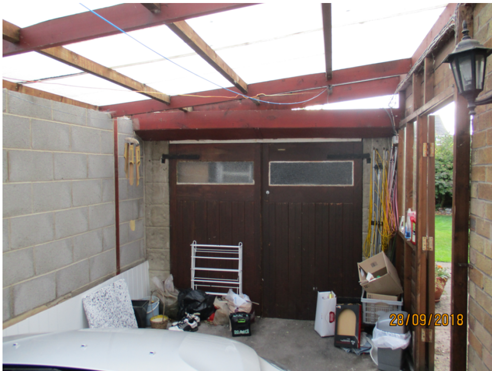
Inside the carport looking towards the applicants garage
